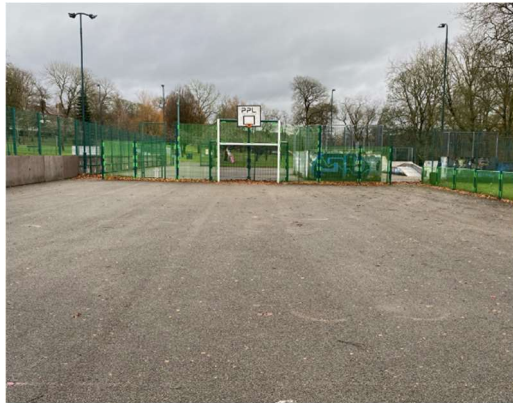
Faded line markings
