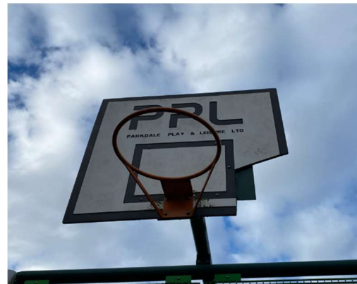
Damaged basketball backboard
