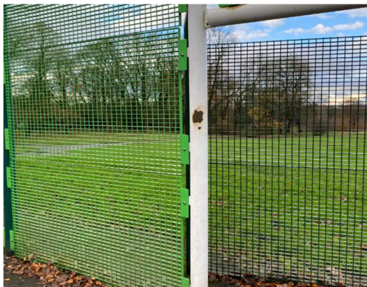
Rust on goal posts
