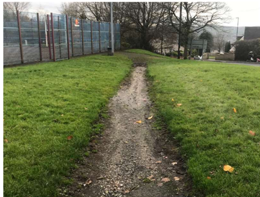
Path connection in poor condition
