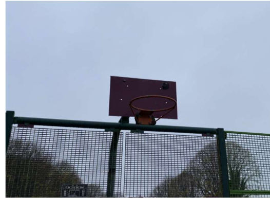
Damaged basketball backboard
