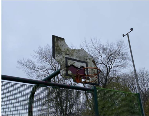
Damaged basketball backboard
