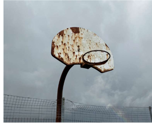
Rusted basketball backboards
