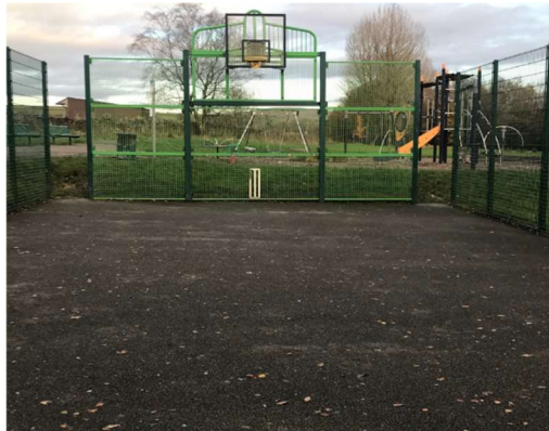
Faded line markings
