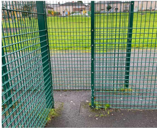
Narrow access restricts disabled use
