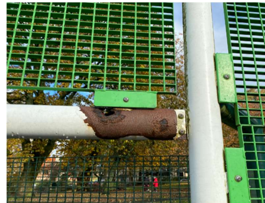
Rusted goal post at fixing
