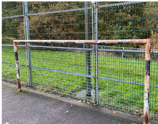
Rusted goal posts
