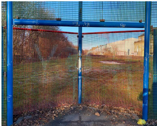
Scuffs/paint missing on goal posts
