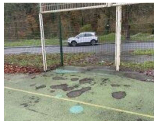
MUGA surface in poor condition
