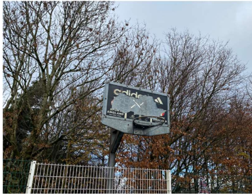
Damaged basketball backboards
